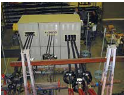
Imoulse Voltage Withstand Test
