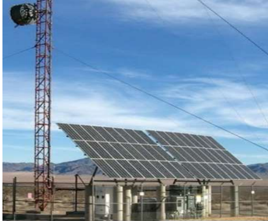
Solar & Wind turbine for BTS
